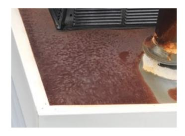
This is a prefabricated fireplace chimney top. You can not see the damage from the ground to the chase cover because to hide the ugly rust they installed aluminum white trim. This will eventually leak cause the fireplace to rust and deteriorate, possible mold growth inside the chase. New chase cover cost \$1800.00. New
