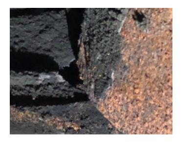
This photo is of a prefabricated fireplace that passed a level 1 inspection from another chimney company. The hole in the collar is a major problem and at this point the unit is not fixable. Estimated cost \$11,000 plus permits
