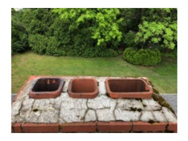
The photo above is of the crown or wash. The cracks are an easy fix now with products designed to seal. Had this gone undetected freeze thraw cycle could have caused this chimney to need a rebuild. Estimated cost to crown coat \$700.00 10 year warranty. Estimate cost to rebuild \$8000.00 10 year warranty.
