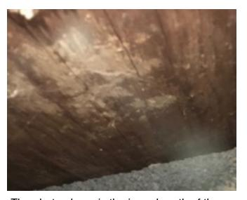
The photo above is the inner hearth of the fireplace( or firebox directly below where you build fires) the under side in the basement. This is a wood form that should have been removed after construction at this point it is too late. This system must be altered to a system that allows combustibles underside of the hearth. Estimated cost \$13,000.00 + permit.
