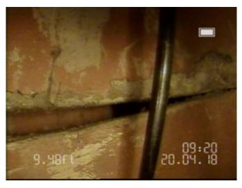
This photo was taken during level 2 fireplace was never use. Has missing mortar between terra cotta liner. A level 1 inspection would not have revealed this defect. This chimney has a metal firebox. Estimated cost to repair \$12,000.00 plus permits
